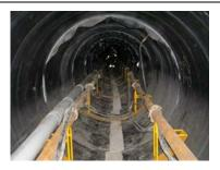
b. Slurry pipes & lubrication lines
